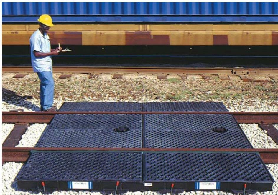
These trackpans have been manufactured specifically for this purpose and fit neatly between, and alongside the existing rails. The units can be connected together to combine their capacity, or can be plumbed to a sump or the adjacent containment via below grade piping.
